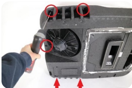
1) Unscrew the roof cover (5 screws)
